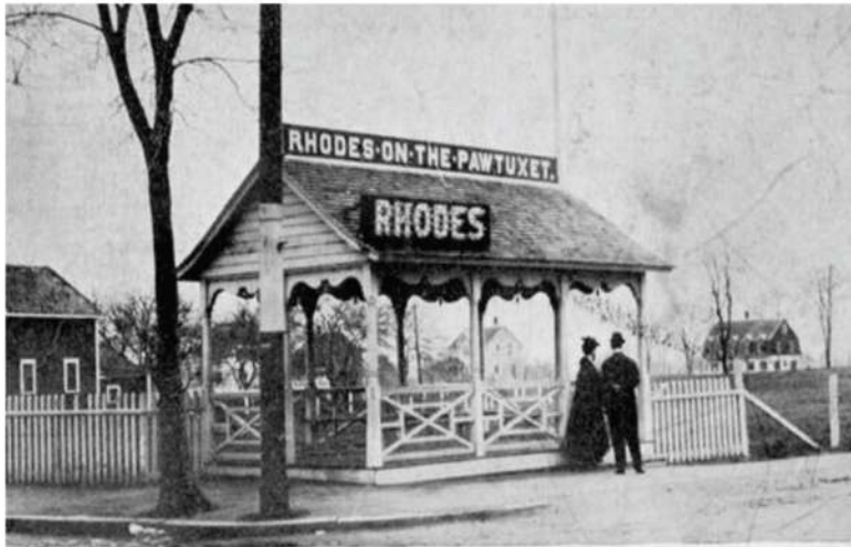
Waiting Station at Rhodes, Pawtuxet, R. I.
