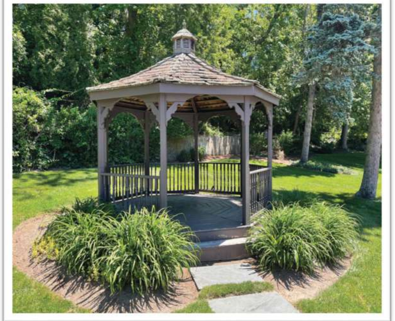
THE STATUE OF TERPISCHORE, MUSE OF THE DANCE, AND THE RHODES GAZEBO LOCATED OUTSIDE OF THE MAIN ENTRANCE TO RHODES. BOTH STRUCTURES SURVIVED THE FIRE, AND WERE ADDED TO THE NATIONAL REGISTRY OF HISTORIC PLACES IN 1978.
